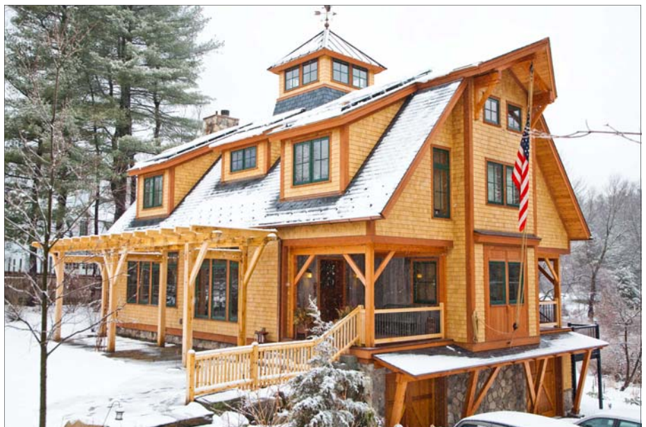
The four-bedroom prefabricated home, received a LEED Silver Certification from the United States Green Building Council for its sustainable design.
